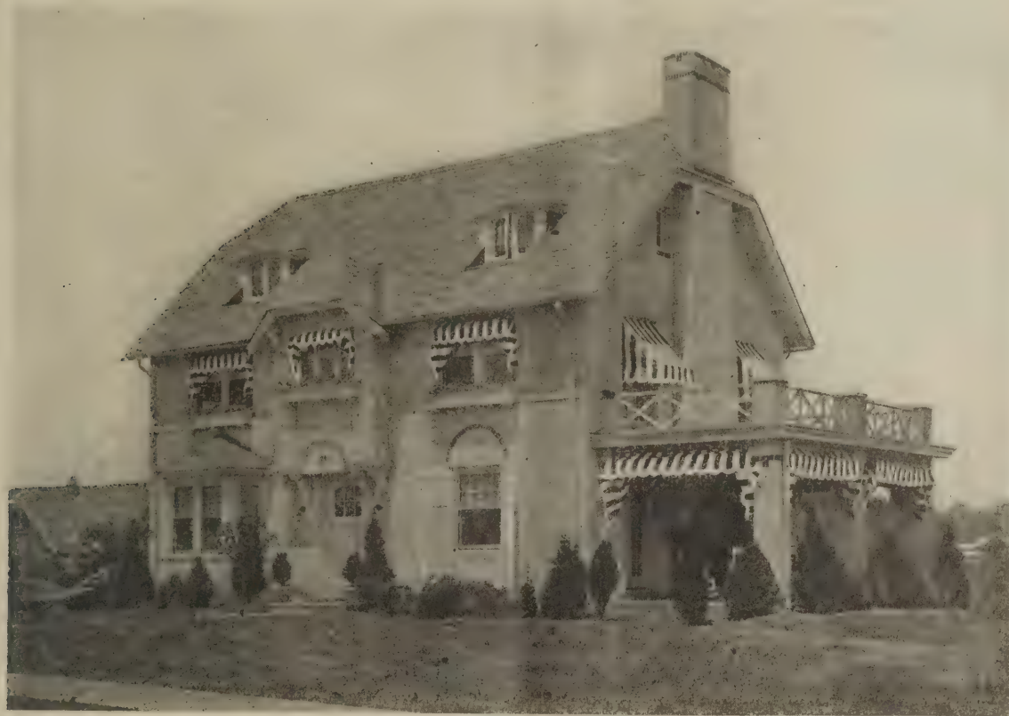
AN ARTISTIC HOUSE CONSTRUCTED WITH WALLS OF STUCCO ON HOLLOW TILE REX STACKHOUSE, ARCHITECT
